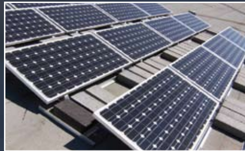
FLAT ROOF BALLAST SOLUTION
